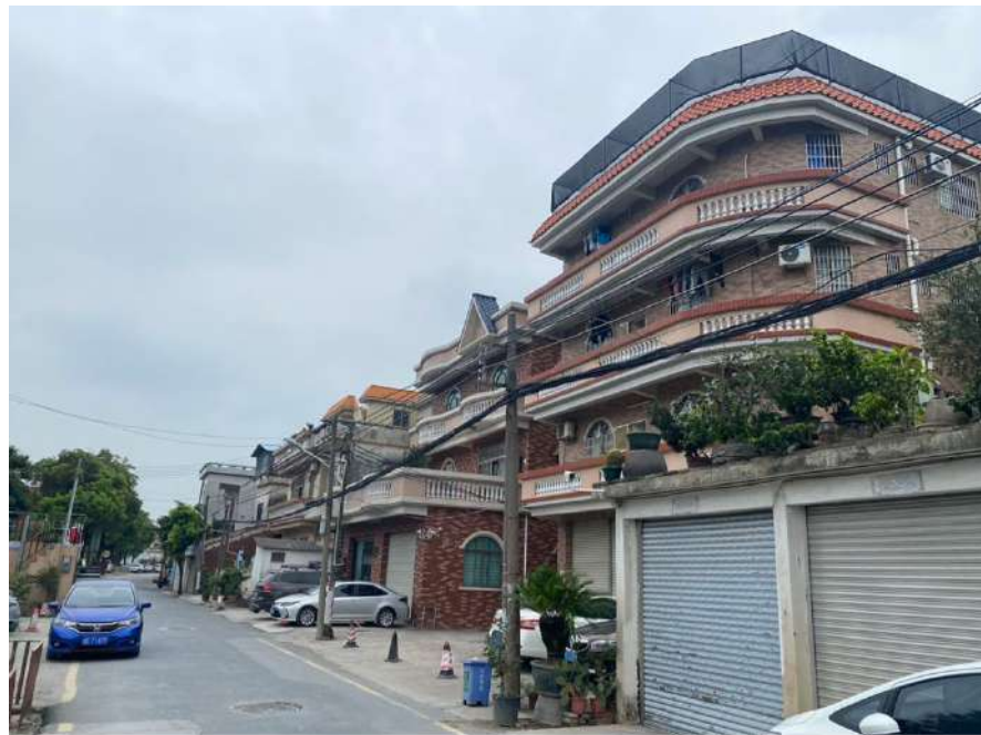
Figure 5. Residential Buildings in Chencun Village, China.
