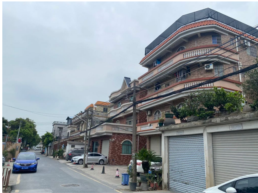
Figure 5. Residential Buildings in Chencun Village, China.
