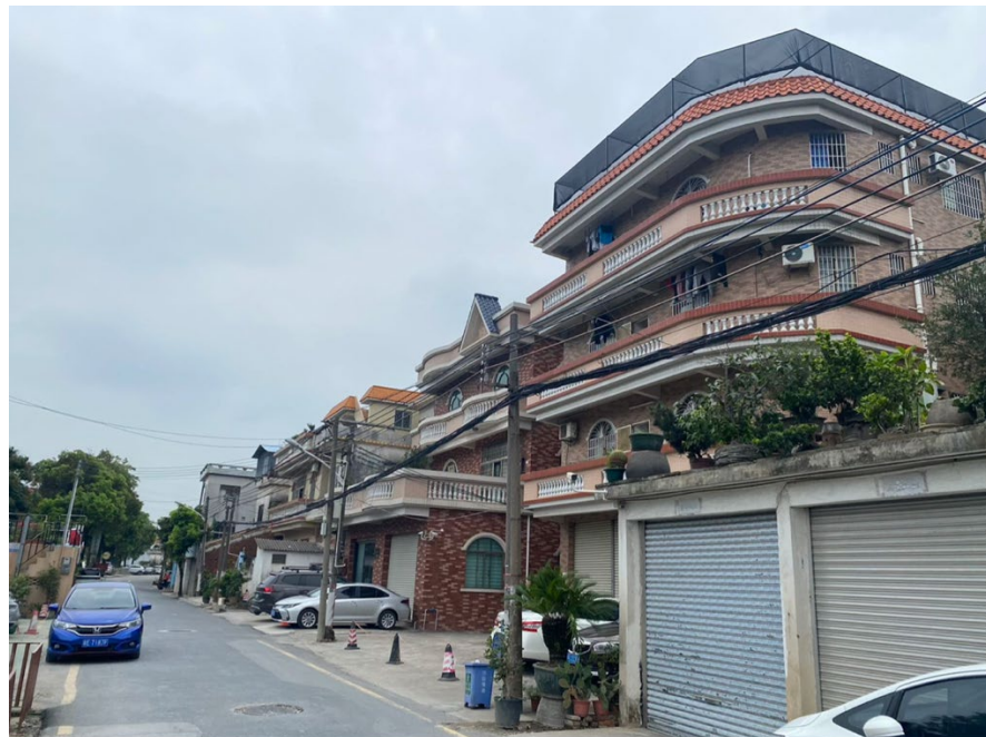
Figure 5. Residential Buildings in Chencun Village, China.
